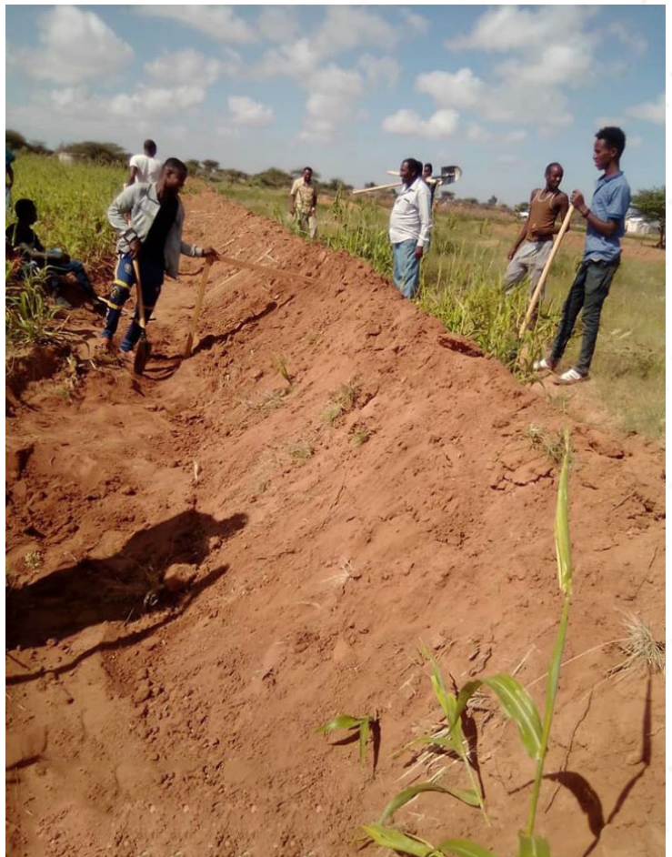
Community members constructing contour bands Soil and Water Conservation
