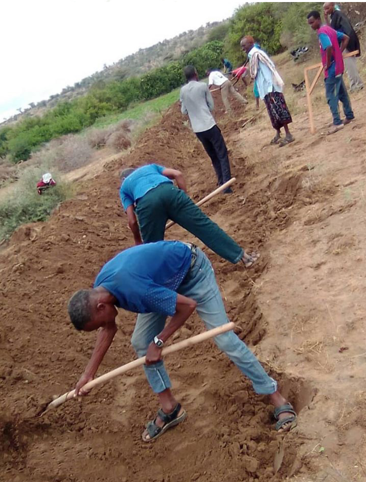
Community members constructing contour bands Soil and Water Conservation
