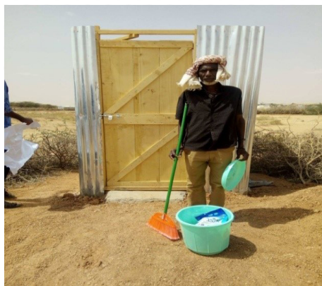
New latrine with cleaning tools, Yirowe
