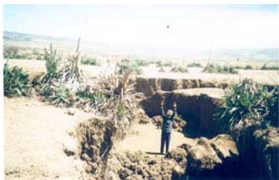
Fig. 3: Gully erosion threatening previous rehabilitation works done before the civil war. Bookh Valley, east of Gacan Libaax
