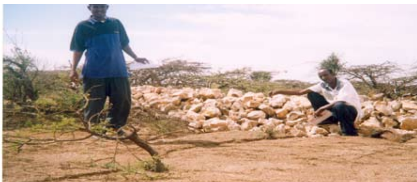
Fig. 20: Rehabilitation work in Gacan Libaax: Rockdams
